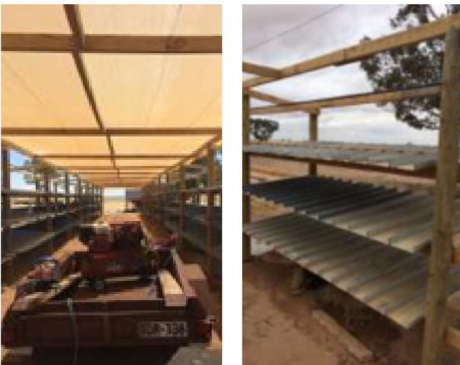
Left - Construction of one bay of trays and (right) a view of the fodder shed with the shade cloth roof.
